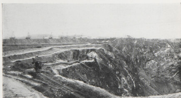
A panoramic view of the vast amphitheatre of the Canadian Johns-Manville mine at Asbestos, which covers an area of 50 acres. It is a shallow mine, and constantly extends as the terraces are cut further back into the rock. Portable railway tracks are laid along the terraces, and dump trains move the broken rock from terrace to mill. When a new terrace is blasted the tracks are moved into the "face". A machine called a "track mover" is gripped to a length of track and in a few minutes it moves the track to the new position, lifting it about two feet at a time, ties and all. In the dim distance, near the centre, is seen a church steeple, a land-mark of the village of Asbestos, which is on the edge of the mine and is gradually being pushed
