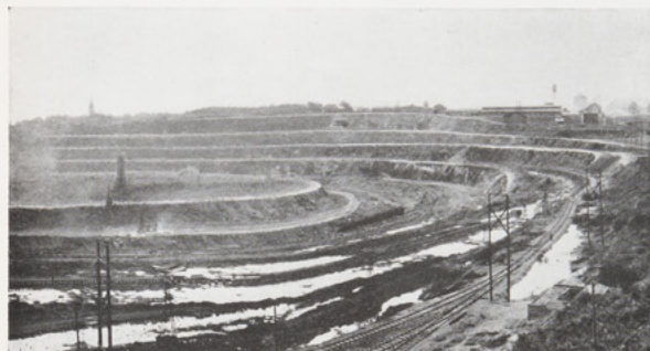
further away by the growth of the mine in its direction. Below is the Asbestos Corporation pit at Thetford Mines. It is a deep mine, being 450 feet from the surface, with the sides rising steeply. The method of moving rock from the working "face" here is by "scoops" which are first hoisted vertically to cable-ways, and then drawn horizontally along the cables to the cable stations, from which dump trucks take it to the mills. This is the greatest cable-way system in the world having a length of 1,400 feet between derricks, and being capable of lifting over 7,000 tons of rock every working day. The Bell pit is seen in the distance.
